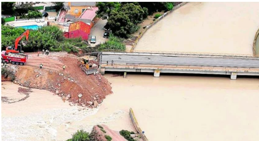
Figure 12. Breakage of the channelling of the river Segura at Almoradí. Source: Segura River Basin Authority.
