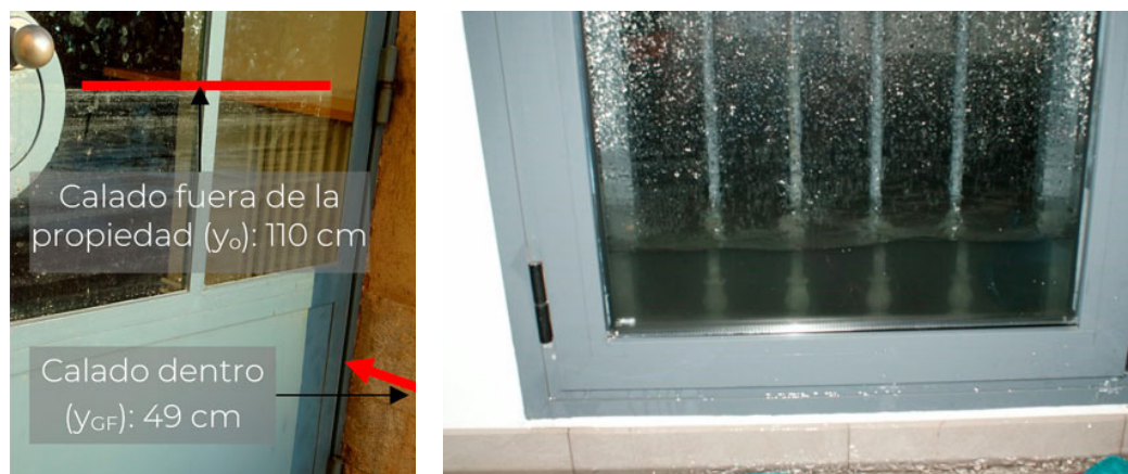
Figure 8. High-water marks following a flood event both inside (49 cm) and outside (110 cm) a property.
