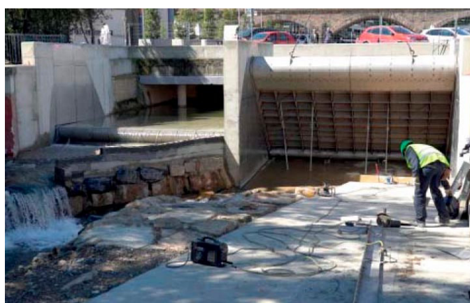
Setting up caissons at the confluence of the rivers Queiles and Ebro. Tudela (NA).
