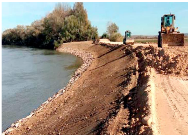
Repair and refurbishment of a dyke in Osera de Ebro (Zaragoza).
