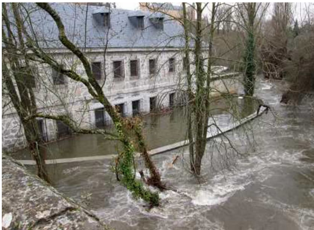
Figure 1. Terrace of the Royal Mint building in Segovia under water during the 2014 flood.
