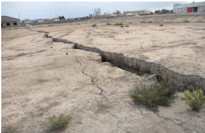
Figure 9. Piping phenomenon at the Los Soles spot in Puerto Lumbreras station.
