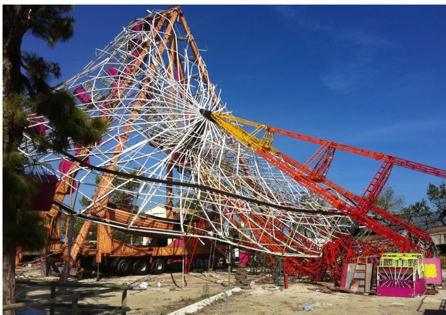
Figure 5. Tornado damage at the Gandía fairground.
