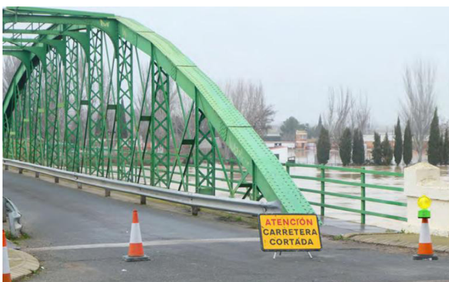
Figure 9. Bridge over the Ebro where it flows through Gallur (Z). Source: CCS.
