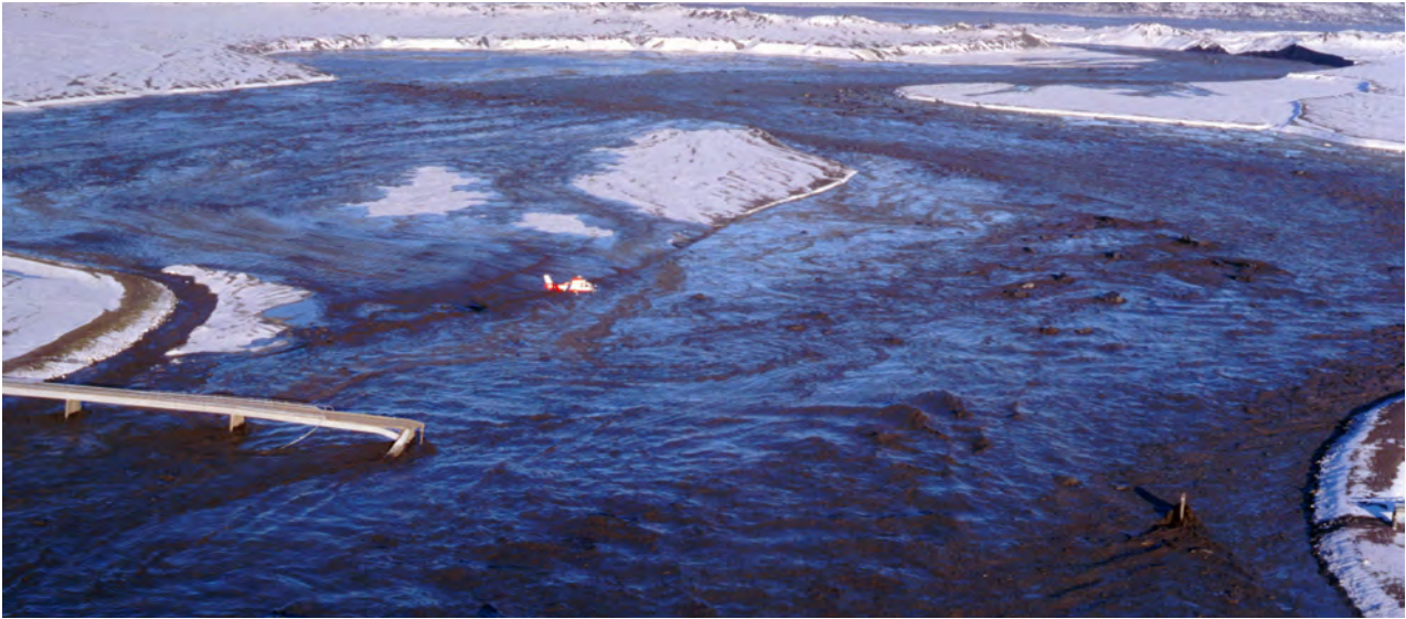
Figure 3. The jokulhlaup resulting from the eruption in Gjalp in 1996. The bridge was destroyed by the large icebergs carried with the floodwater.
