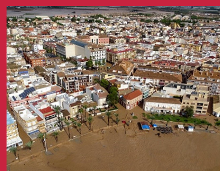
Figure 1. Flooding in Los Alcázares (Murcia) in September 2019.
