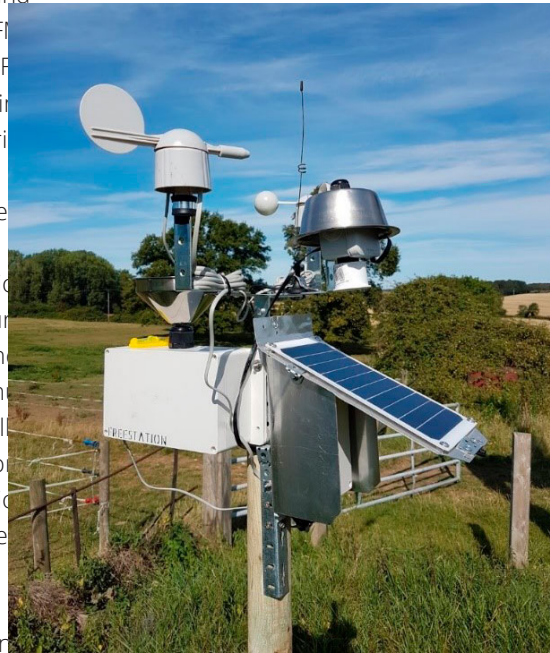
Figure 2: Image of a //Smart:River FreeStation: using IoT for flood prevention.
