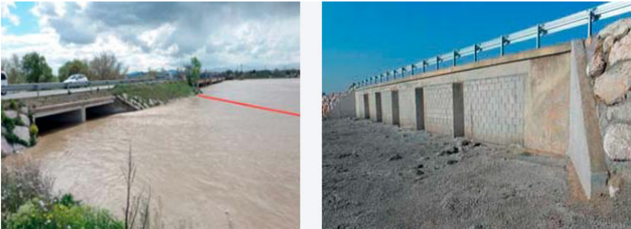
Frames on the river Ebro next to the CV-04 bridge in Novillas (Zaragoza) and integrable frames on the A-1107 road. Pina de Ebro (Zaragoza).
