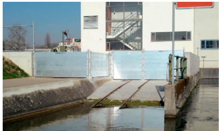
Figure 6. Example of resilience measures in buildings: Watertight modular closing doors in enclosing walls.
