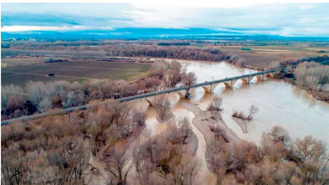
Curage in Alfaro (La Rioja) after the action of a flood on the River Ebro.
