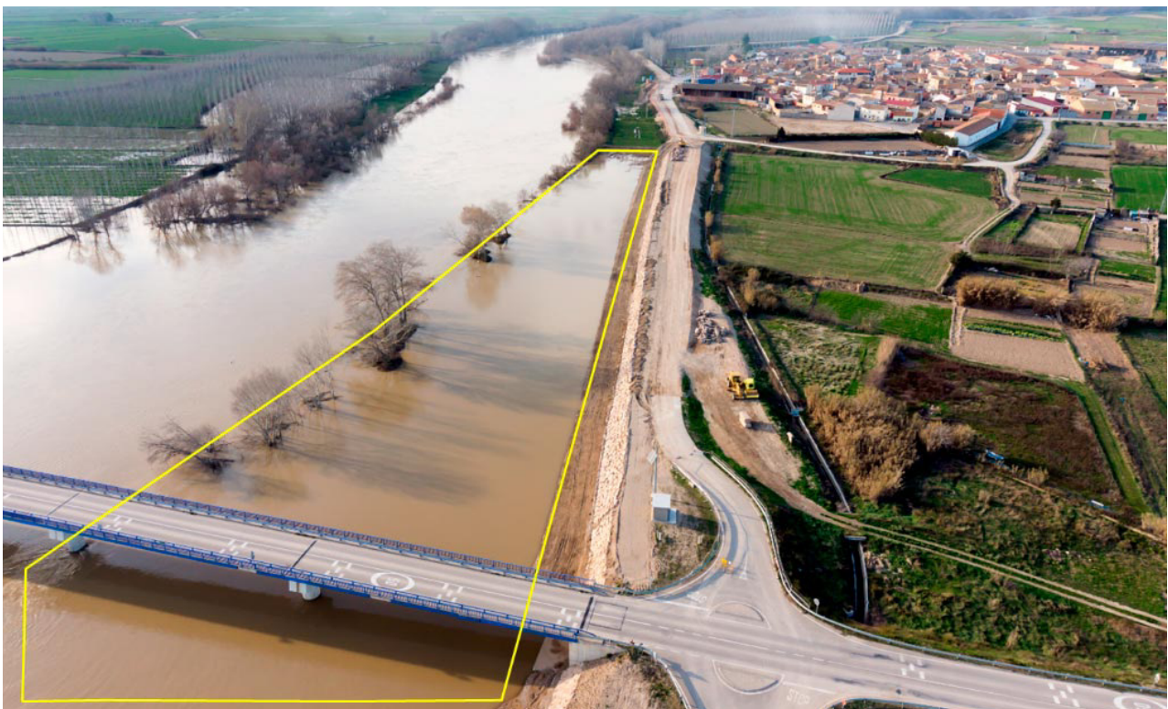
Pradilla de Ebro, increasing the permeability of the bridge over the river Ebro.
