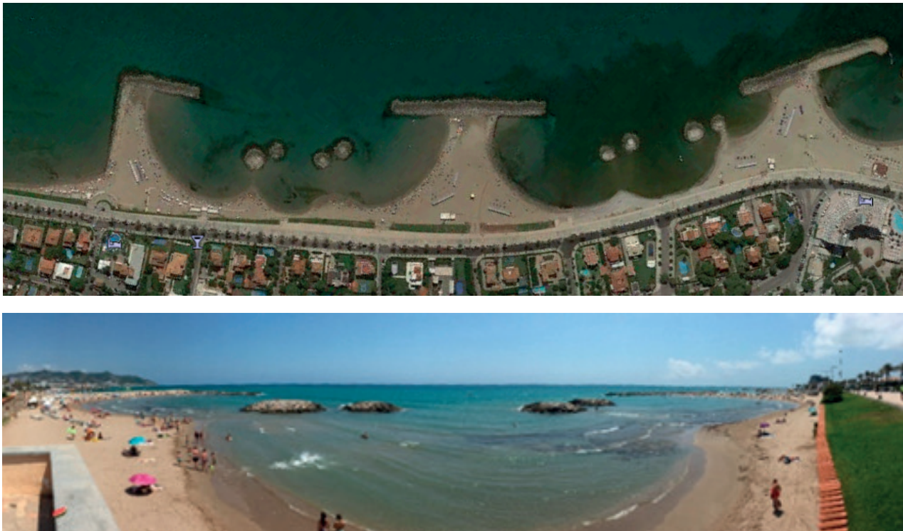
Figure 4. Beach stabilised using a system of dykes and seawalls. Sitges (Barcelona).
