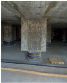
Photograph 1. Example of a seismic insulator
