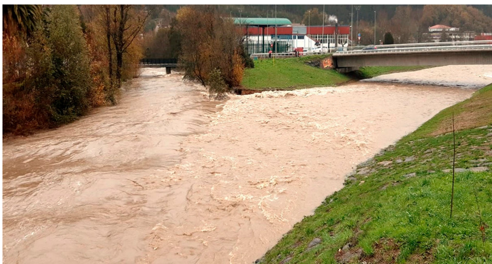
Figure 9. The Cadagua River during a flood with the recovered floodplain acting as an additional channel.
