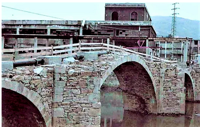
Figure 3. The Mercadillo Bridge in Galdakao after the August 1983 floods. The height attained by the water is clearly visible. Source: Biscay Provincial Council, 1984: "Torrential rains. August 1983. Quantifying the Disaster".
